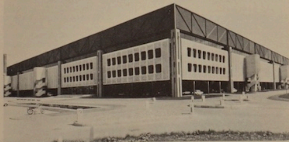
Bovis Construction Division was awarded a Management Contract worth £7½ million to supervise the building of the John Player Horizon Factory at Nottingham. The two storey factory occupies a 30 acre site and its power supplies are generated totally by Natural Gas. The whole building programme - from initial planning to completion - took just 31 months.
