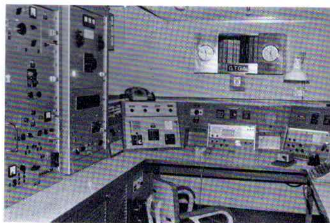
Radio Office watchkeeping position
