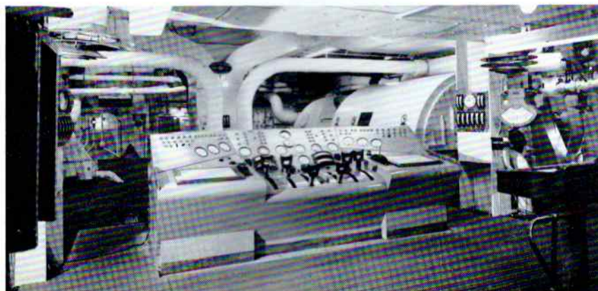
ENGINE ROOM STARTING PLATFORM
