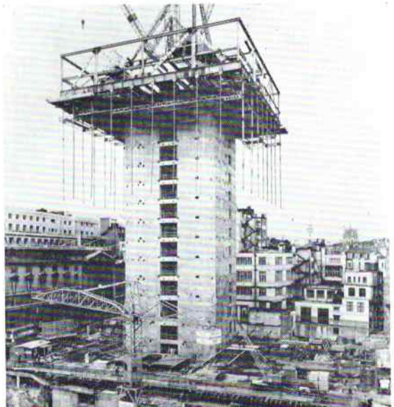
Core completed, the hanging structure begins.
