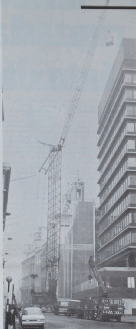
The transformer being lowered on to the roof of the P & O Building
