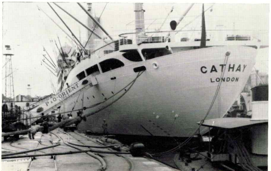
'Cathay' transferring water to the reservoirs at Hong Kong
