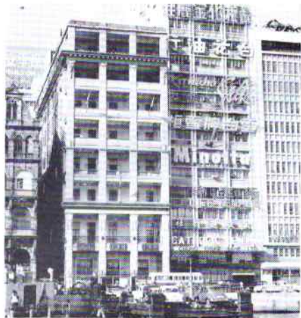
Former P & O Building, with the Catholic Centre towering over it.
