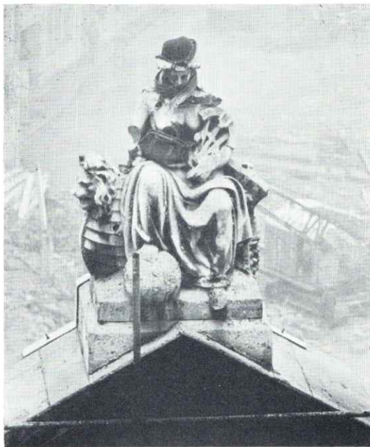
'122' The figure of Neptune which crowned the entrance to our old offices was removed with some ceremony. The demolition workers clothed the old gentleman with some sort of garment and what looked like a bowler hat.
