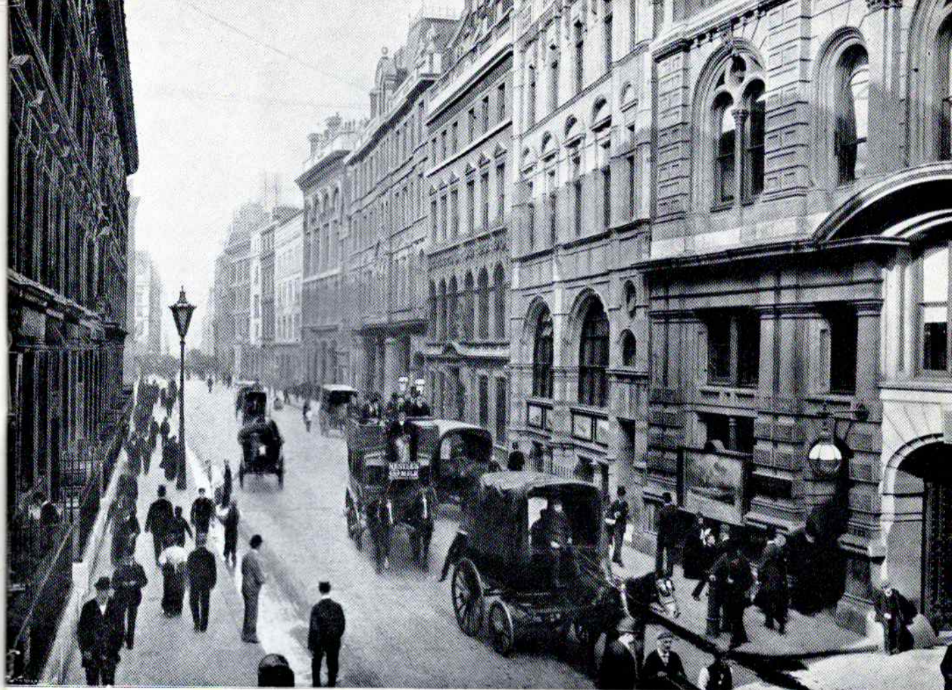
Leadenhall Street in 1898, showing the P & O Offices on the right, looking very much as they do today.
