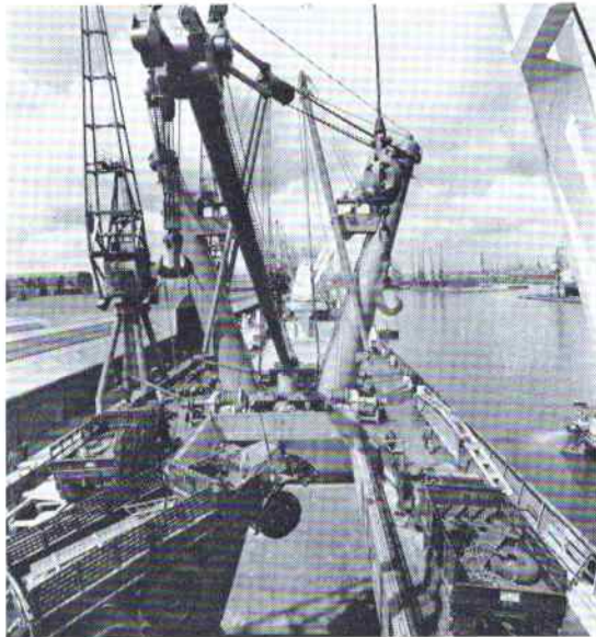
A view from the bridge showing the heavy lifting gear.
