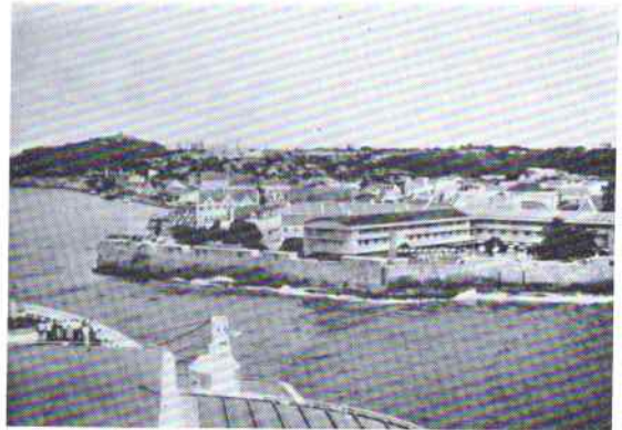
The vessel coming nicely into position to enter the channel.
