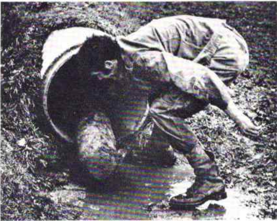
A sewer caused little trouble. The first cadet emerges and pulls whilst his colleagues, inside, push.
