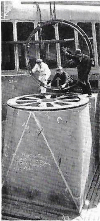
"Oriana" is fitted with eight 5-ton A.S.E.A. cranes. The base ring for the port crane to No. 3 Hatch is seen being lowered on to the crane plinth.
